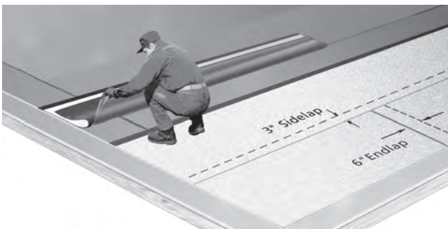
Figure 5-21: Once positioned, lift and fold back the lower half of membrane.
