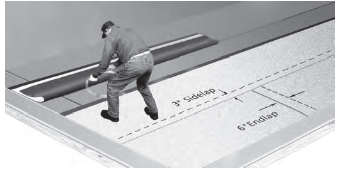
Figure 5-22: Remove the selvage edge release strip.
